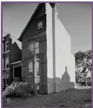
Terrell House (Library of Congress)
